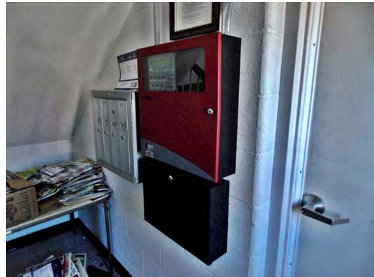
One of the common fire alarm control panels within a residential building.
