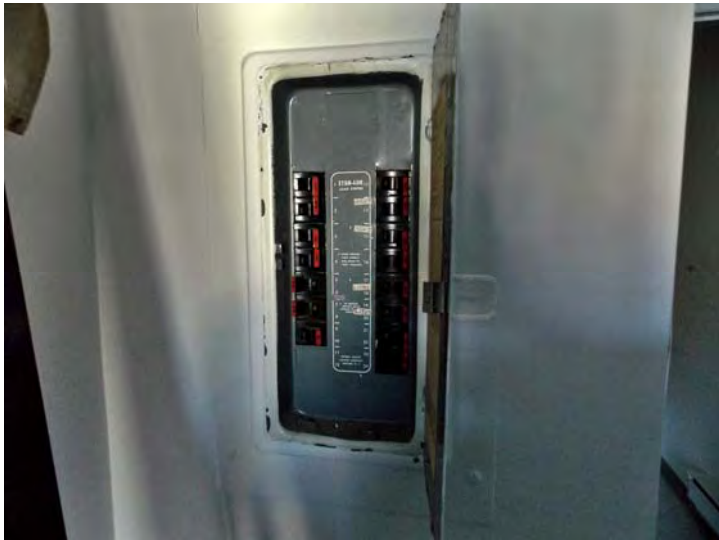
An example of a Federal Pacific (FPE) Stab-Lok circuit breaker panel.
