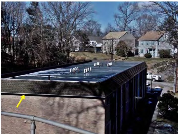
Building D has a rubber membrane roof covering. All buildings have a mansard (arrow) of asphalt shingles.
