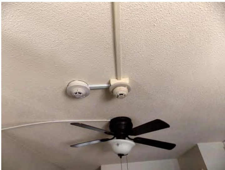
In a few cases, a newer smoke detector has apparently been added adjacent to an older one.
