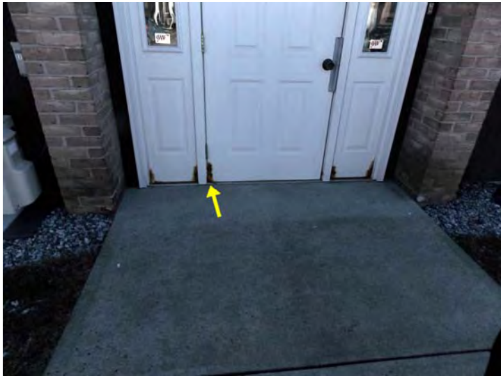
Rust was observed along the base and frame of common entrances.
