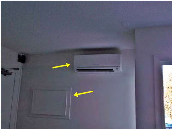
A heat pump terminal unit (upper) and a close-up air conditioner sleeve.
