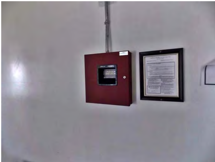
This is the fire alarm control panel that serves the community building.
