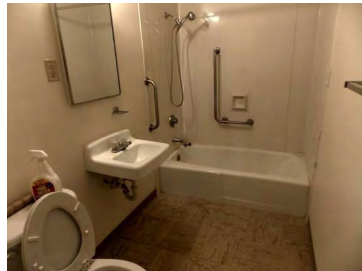
Bathrooms include wall-hung sinks, VCT flooring, and fiberglass tub surrounds.
