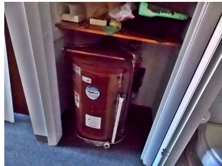
Each apartment has its own electric DHW tank.
