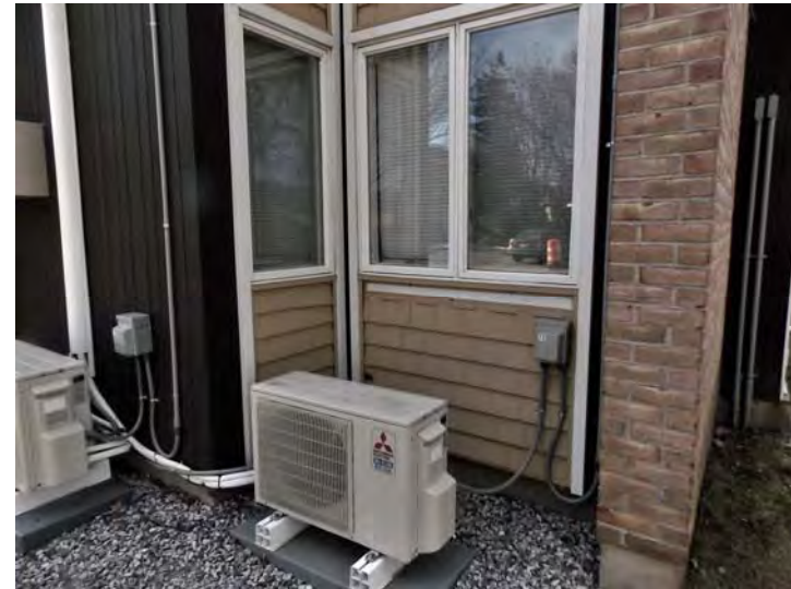
One of the heat pump condensers.
